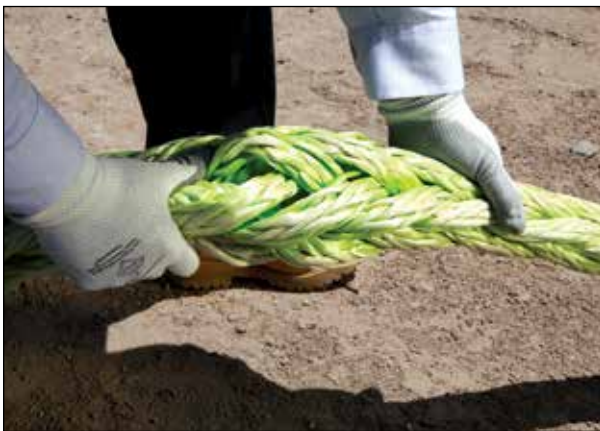
“Hand-compress” the braid at the affected area to open up the construction.
