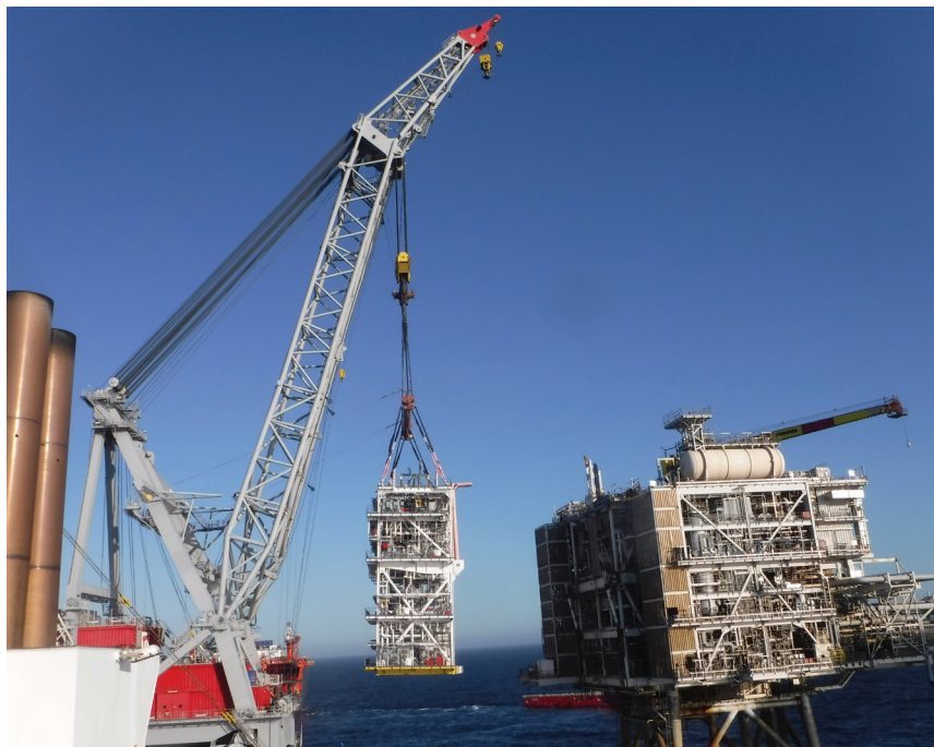
Positioning the 800 tonne topside module
