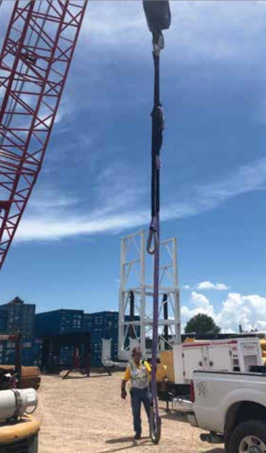
When load handling heavy equipment becomes a challenge—especially when lifting loads with differential sling lengths—adjustable high performance synthetic rope slings are ideal tools. Cortland offers high performance synthetic fiber rope slings in an adjustable form: Extender™ Slings.
