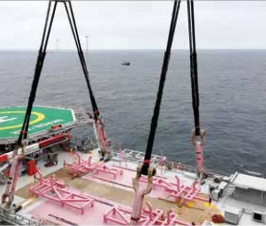
High performance synthetic round slings are as strong as steel wire rope slings, yet light weight, and are safer and less labor intensive. Even the heaviest of loads can be quickly and safely rigged and lifted, minimizing downtime.
